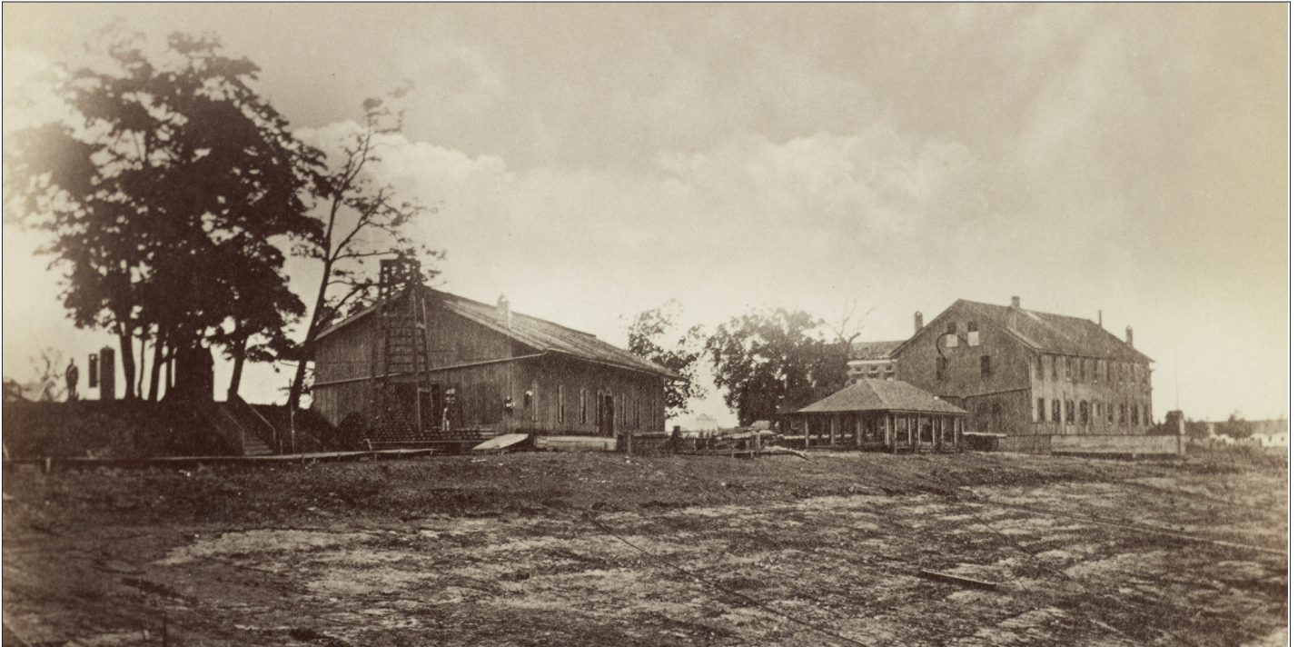
Part of the naval station stands beyond the marine ways at Mound City, circa 1864. The marine ways allowed steamboats to be hauled entirely out of the Ohio River, enabling shipwrights and carpenters to repair and improve them for wartime duty. A marine stands on guard by a sentry box at left. The building next to him may be the original railroad depot. The large brick building seen through the trees in the distance may be the hospital established in 1861, and which accommodated both Union and Confederate wounded pouring into the city in the wake of battles at Shiloh, Vicksburg, and elsewhere. Library of Congress (Control No. 2013647551, LC-DIG-ppmsca-34045).
