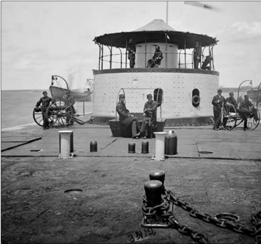
Officers and crew of Catskill with boat howitzers at Charleston Harbor. Lieutenant Commander Edward Barrett sits atop the turret in front of the pilot house. The view shows indentations from battle damage on the turret, as well as how the XV-inch Dahlgren gun could not fit through the porthole in the turret. Glass negative, 1865.
