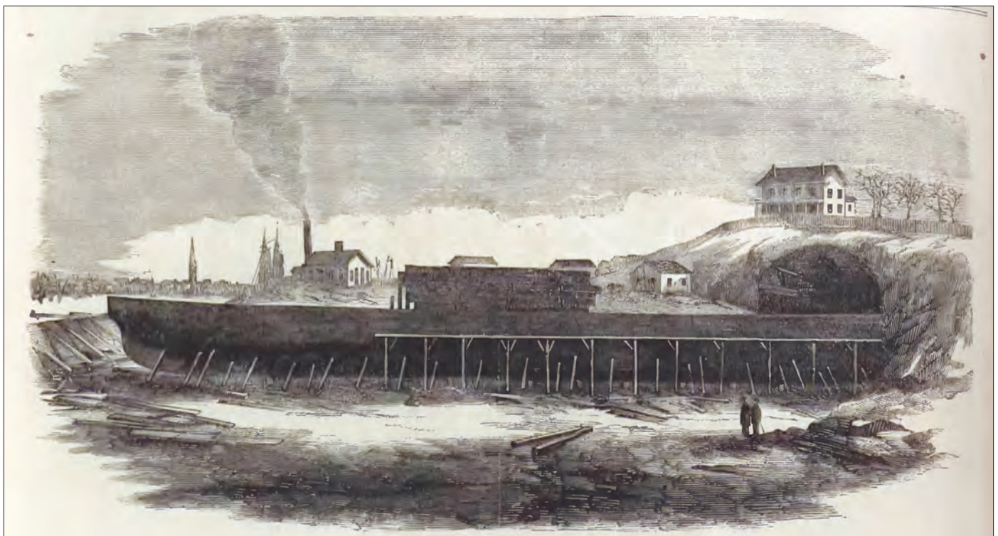
Stevens's Bomb-Proof Floating Battery. Illustration based on a sketch by B.S. Osbon published in Harper's Weekly , Volume V, No. 227, p 284, May 4, 1861. Osbon reported (reprinted from the World ): "...It is said, when completed, there will be nine shells or plates of iron, with space between, making a wall twenty-seven inches in thickness. Being sharp at the bow, she can be used for cutting a vessel in two. She was designed to carry thirty guns of the heaviest caliber on her gun-deck, and mount four Paixhan guns on her spar deck, and furnaces for heating red-hot shot were to be placed in different parts of the ship. Thus built, she would prove a valuable acquisition to our harbor defenses. She will have no masts, and will probably be about 6000 tons burden." ( Harper's , p 285).
